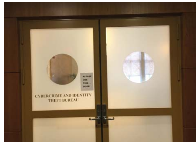
Newly Renovated DA Office Entry
