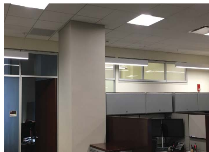
Newly Renovated Open Seating
