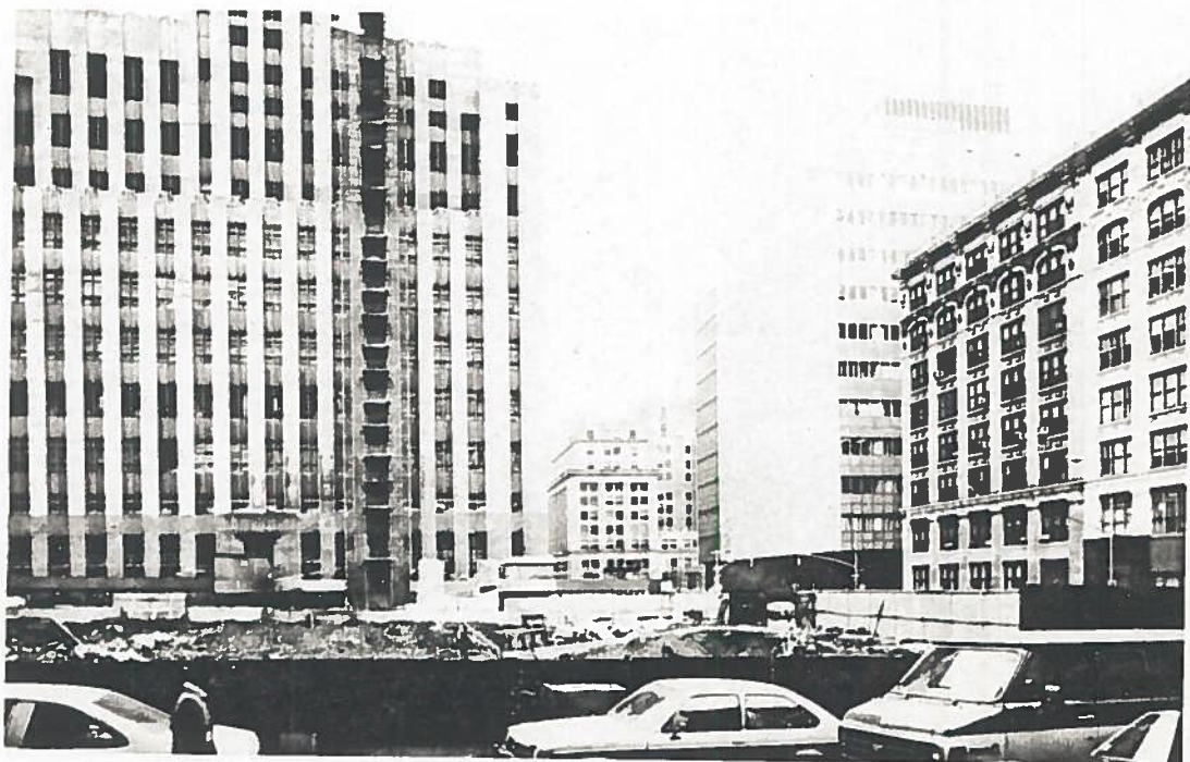
View from Walker Street
